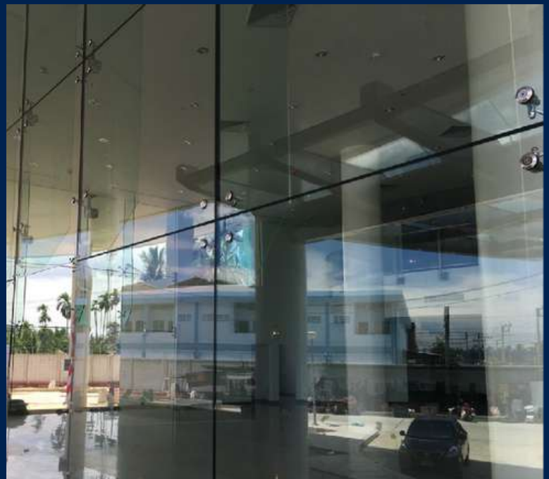
Heat Strengthened Laminate Glass
