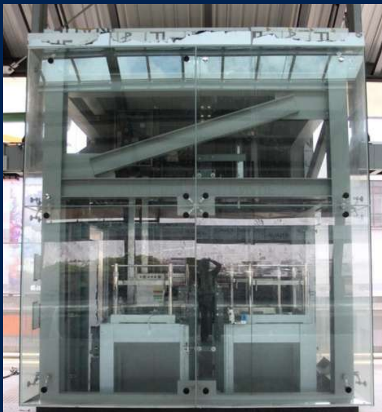
Heat Strengthened Laminate Glass
