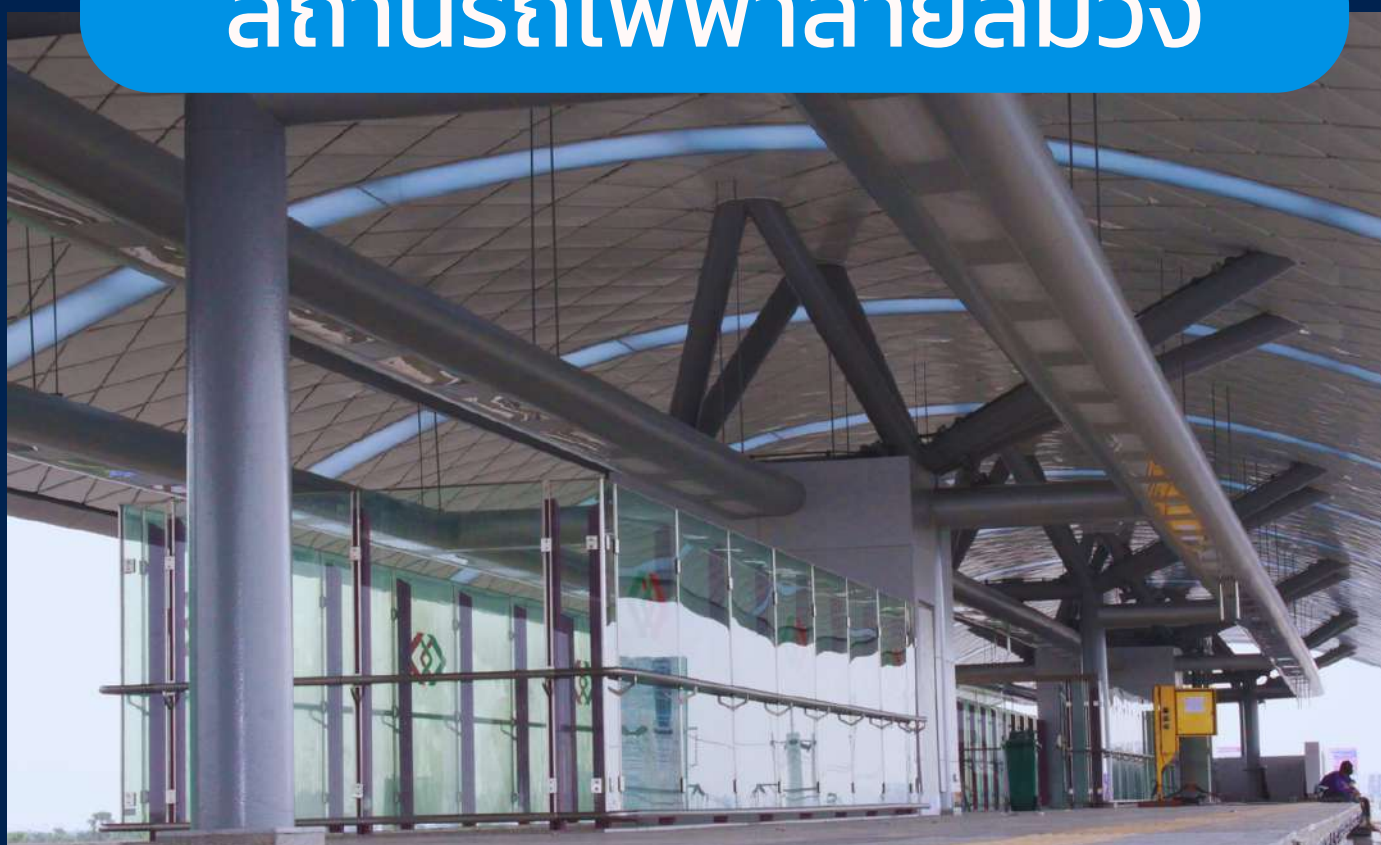
Heat Strengthened Laminate Glass
