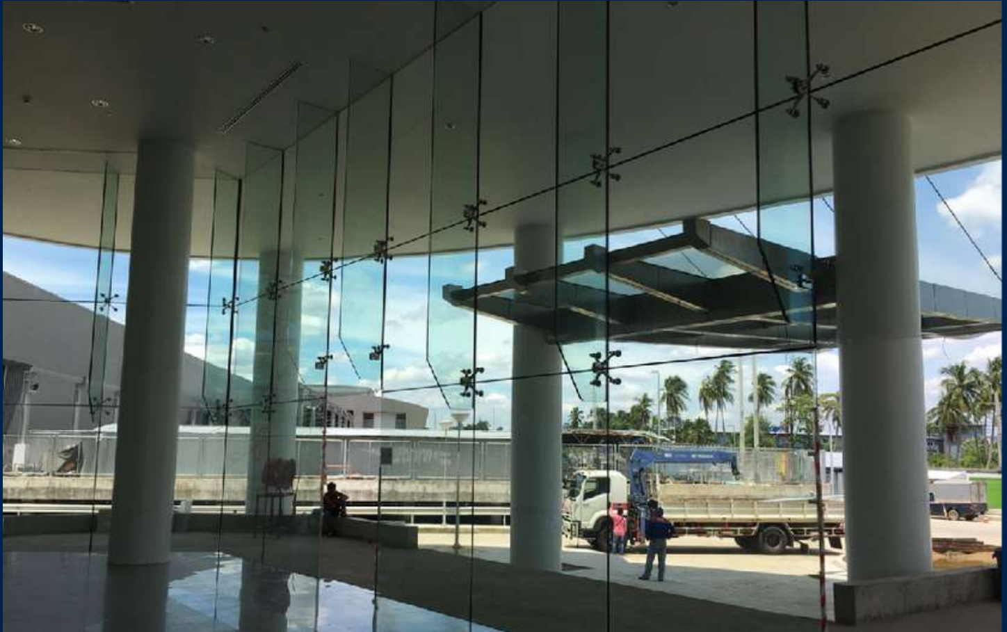
Heat Strengthened Laminate Glass
